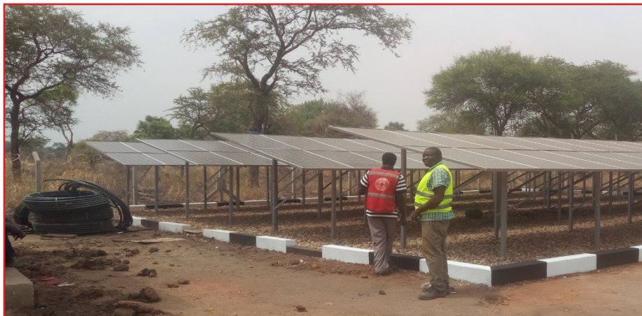
Figure-1: Solar power supply bed consists of 152 solar models of 260W each, for a multi-billion hybrid motorized piped water supply system in Palorinya settlement Zone 3 West.
