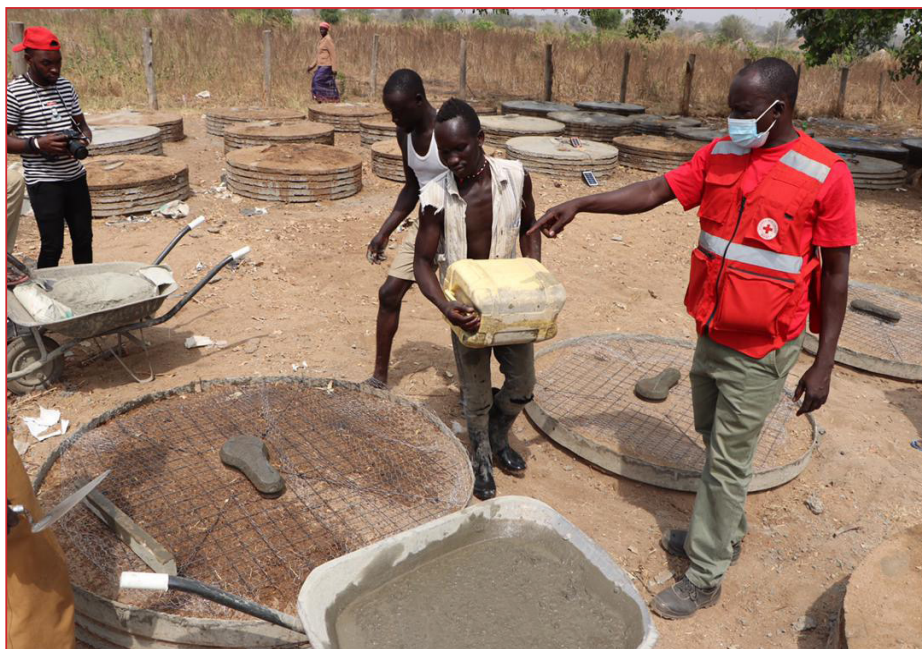
Doom slab productions for construction of the community latrines, the technology which is environmental friendly
