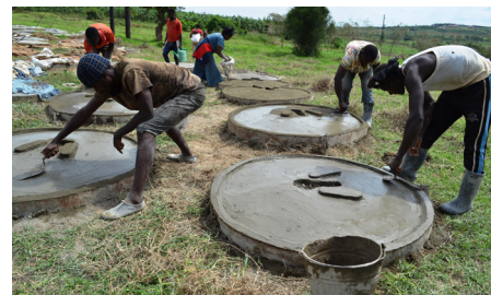
Pit latrine slabs being made under Malteser-Nsamizi partnership for the WASH project in Nakivale refugee camp.
