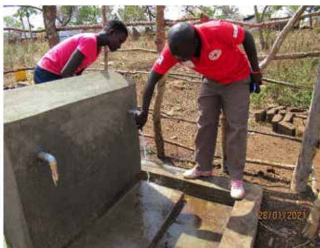
Figure 7: Installed taps at a new tap stand in village 11 which is now receiving water (Jan 2021)
