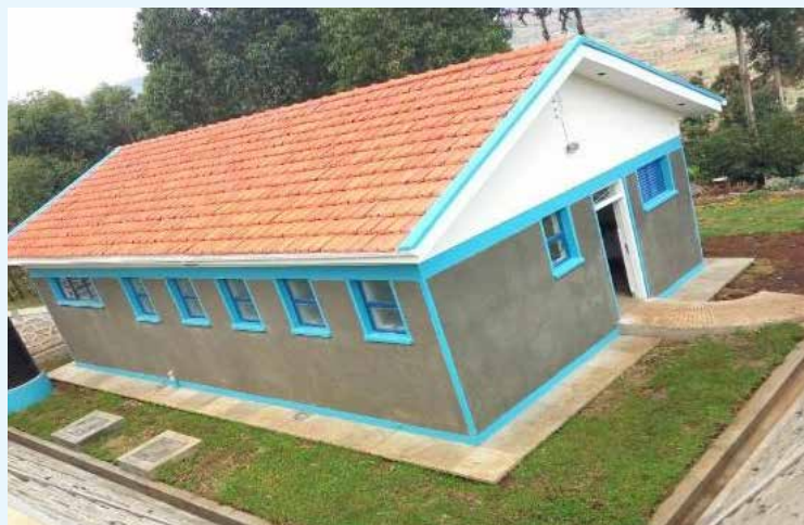
TULEL sanitation facility in Bukwo district.
