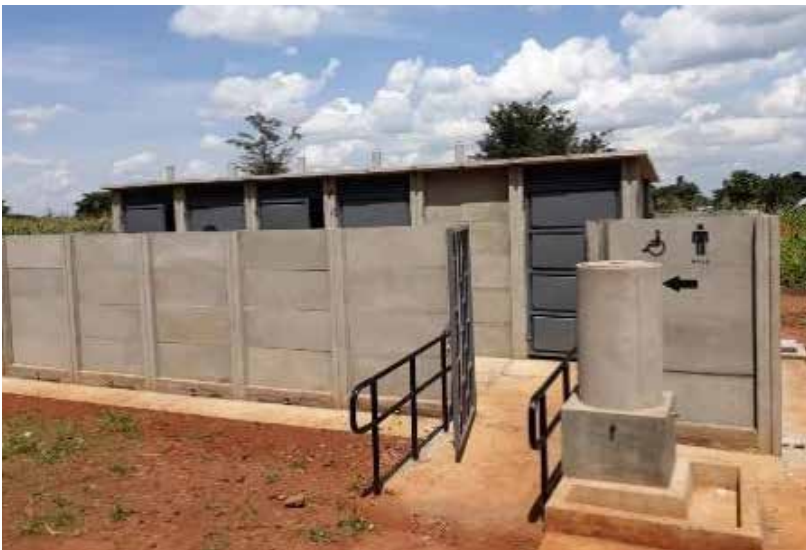
Completed sanitation facility at Kamdini Primary School in Oyam District
